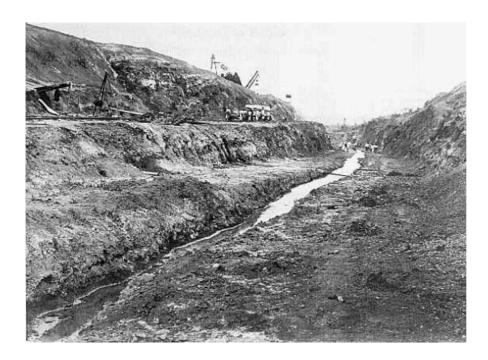
This photograph taken in 1898[1] shows the physically demanding excavation works, needed to cut the artificial valley through the continental divide in Panama.
