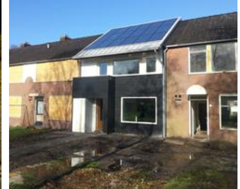
Dutch 'Energiesprong' initiative: houses are super-insulated using panel-facades that adhere to or replace external walls.
