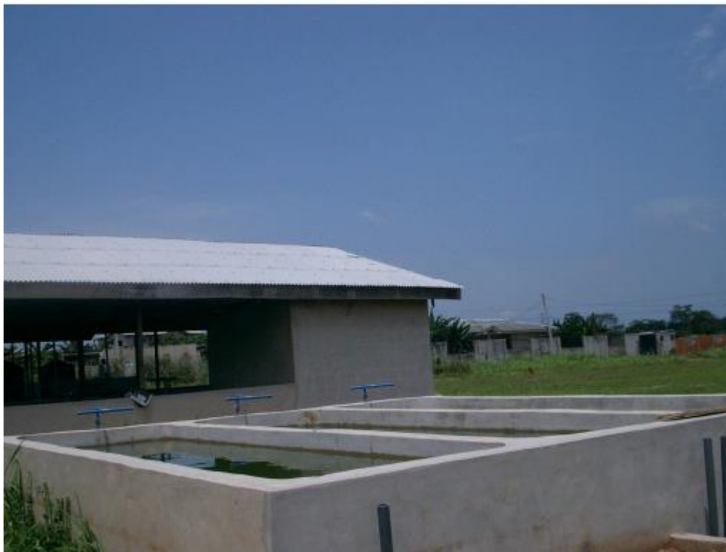
Figure 3:2 A flow-through concrete tank (Fakoya et al. , 2009)
