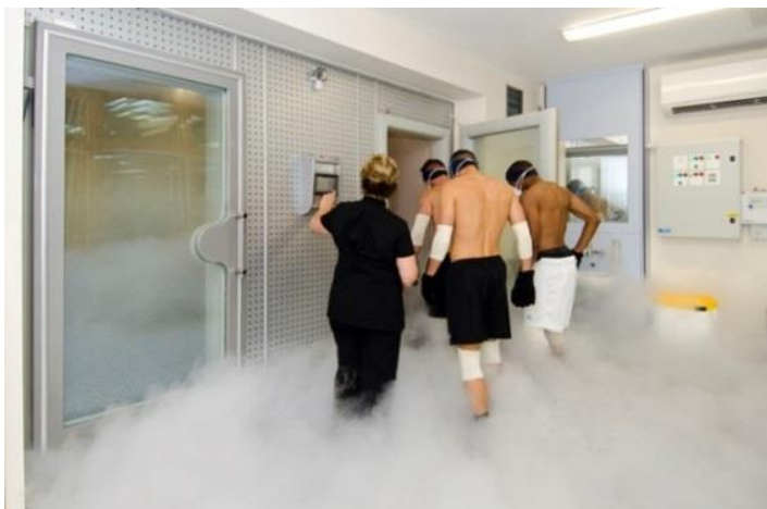
Figure 2.1.1: An example of a whole body cryogenic chamber treatment (Chris Moody Rehabilitation Centre, Moulton, Northamptonshire), typically utilising liquid nitrogen as the coolant, with temperatures set at -110°C to -140°C
