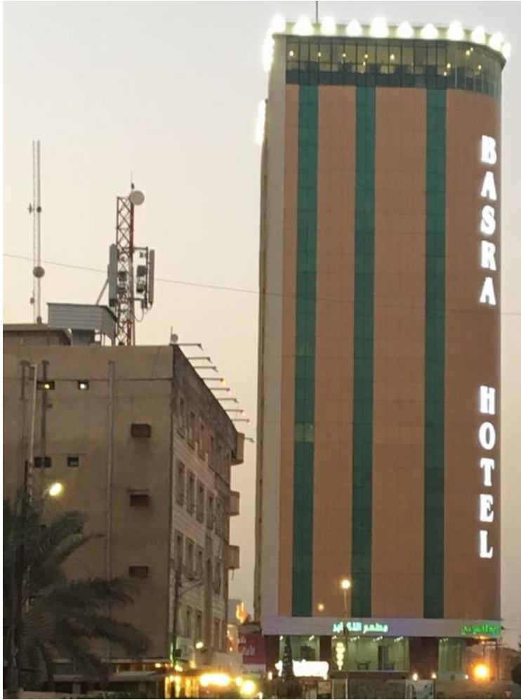
Figure 4.4 – View of the centre of Basra looking onto the Basra Hotel (Researcher, 2017).
