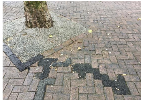
Picture 4: Poor repairs
